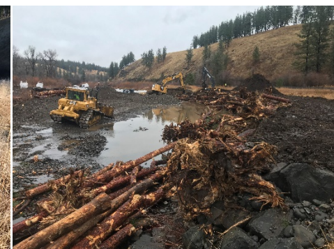
Mainstem Grande Ronde River Longley Project – mainstem pool grading and large wood complexity
